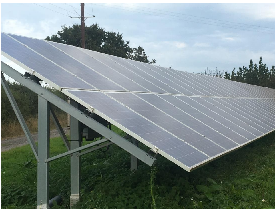
Plate 3-3: Solar Panels with Fixed South Facing Configuration
